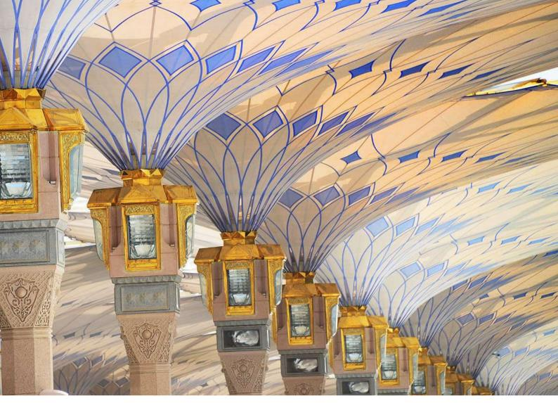
All of our fabric structures are robustly constructed, fully engineered, and permanent to offer years of practical and stunning outdoor protection from the natural elements. We can offer a wide array of fabric options, running the gamut from silicon coated woven glass fabric to an architectural grade PVC.
