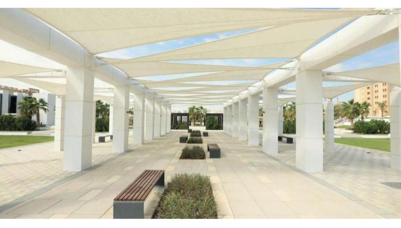
We aspire to produce world-class Tensile Shades structures, which are kept relatively light in weight by deriving their structural stability from their pre-stressed shape, instead of the mass of the material used.
